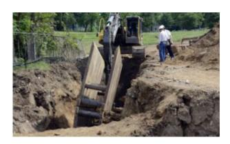
An underground utility crew was installing a water pipeline when a worker entered a portion of the straight cut trench that was about 3.9 metres deep. The trench wall caved in onto the worker. The worker, who was extracted by the crew and transported to the hospital, sustained permanent life-altering injuries. The owner of the excavation company pleaded guilty to violating Sec. 2(2)(a) of the OHS Act and was fined \$30,000 [Vincent Bishop, Govt. News Release, Jan. 10, 2017].
