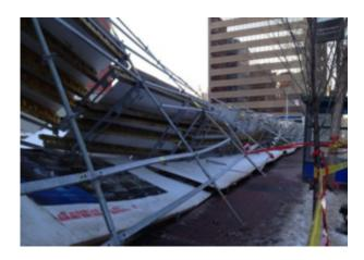
Scaffolds are common equipment and are used to allow workers to safely access and work at areas at heights. But if you build scaffolds incorrectly or use the wrong materials, these structures can be unsafe.
