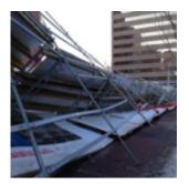
Scaffolds are common equipment and are used to allow workers to safely access and work at areas at heights. But if you build scaffolds incorrectly or use the wrong materials, these structures can be unsafe.
