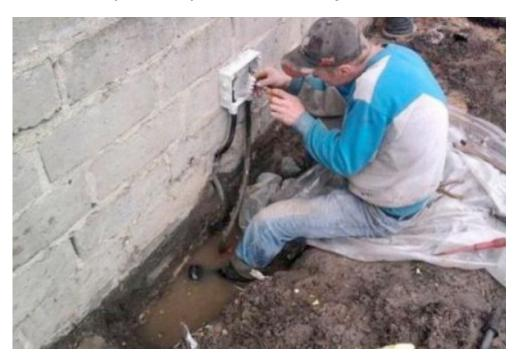
You don't have to be an electrical engineer to recognize that it's not a great idea to repair electrical equipment with one's feet immersed in a puddle. The worker in this picture was fortunate to survive the experience but others haven't been so lucky.
