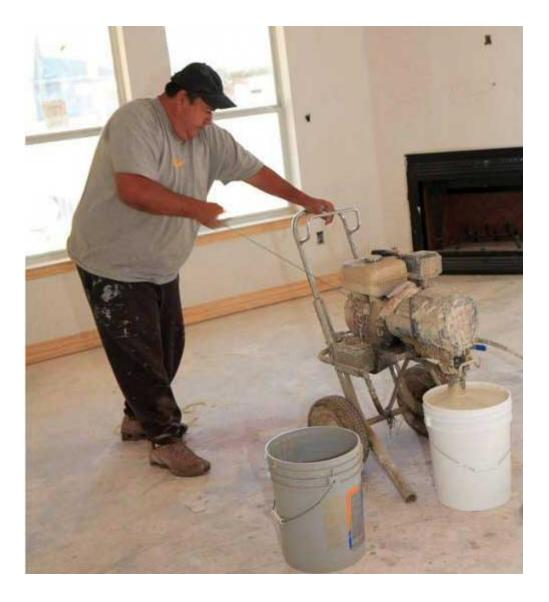
Gasoline-powered equipment, such as the mixer the painter in the photo is using, shouldn't be used indoors. Operating such
