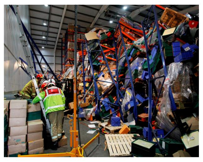
Workplaces such as warehouses, distribution centres and manufacturing plants regularly use racks to store materials, goods, etc. Storage racks help keep the workplace clean and organized, and allow for the safe movement of workers and mobile equipment. But if racks aren't installed and used correctly or are
