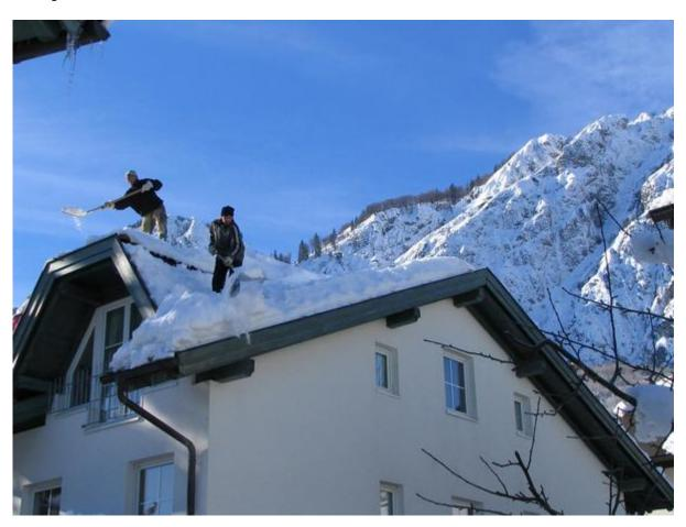
Falls from heights, such as roofs, are one of the most common safety hazards. Roofs are especially hazardous when they're covered with snow and ice, like the roof in this picture. So it's even more important for these workers to be using appropriate fall protection.
