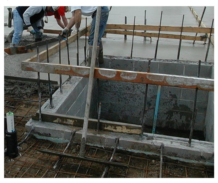
Unguarded protruding steel reinforcing bars ('rebar') are very hazardous. Even if you simply stumble onto a piece of an unguarded rebar on the same level, you can impale yourself'resulting in serious injuries or death. And falls from heights onto uncapped rebar are even more likely to end badly.
