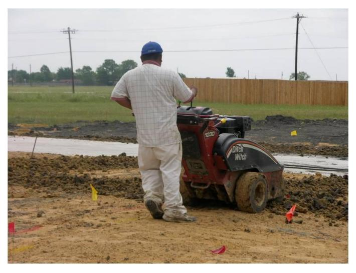
PPE is designed to protect workers from hazards they can see, such as sharp edges or falling objects, as well as those that are invisible, such as excessive noise. This worker should be wearing hearing protection while operating loud
