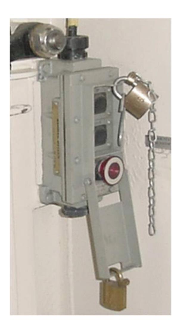
Electrical equipment poses serious safety hazards to workers who have to repair or maintain the equipment. That's why equipment should be powered down and locked out before workers do such work on it. The purpose of the locks is to prevent another worker from powering or starting the equipment.
