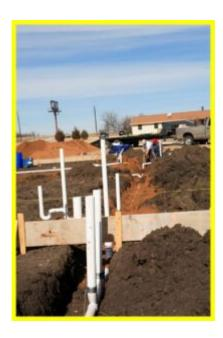
Are these piles of excavated material a safe distance from the edge of this trench'
