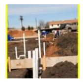
Are these piles of excavated material a safe distance from the edge of this trench'
