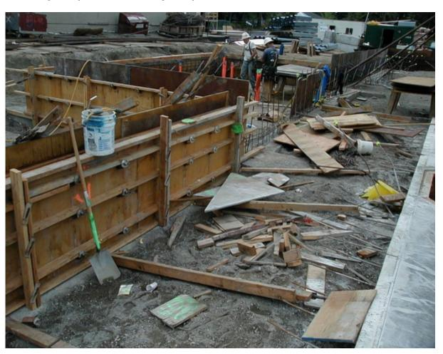
Construction sites can present many hazards to workers, from the mobile equipment used on site to trenches and excavations. But something as seemingly benign as a piece of lumber left on the ground can also be hazardous because workers can easily trip on it and get seriously injured. That's why good housekeeping practices at construction sites'and in other workplaces'are
