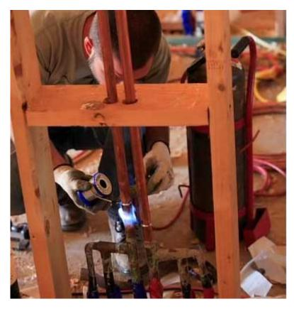
Keeping work areas clean isn't just about neatness. Cleaning up the workplace also eliminates safety hazards. Here, the floor surrounding this worker is covered with wood chips and shavings, flammable material that could easily be ignited by the welding torch he's using.
