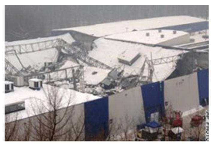
This winter, make sure you clear snow and ice off of the roofs of your workplace facilities. A lot of snow, particularly if it's heavy and wet, can compromise the roof's structural integrity and result in a collapse.
