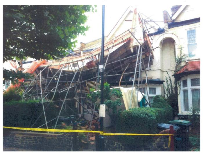
When built correctly, scaffolds are generally safe for workers to use. But even a well-constructed scaffold can become hazardous if it's overloaded.
