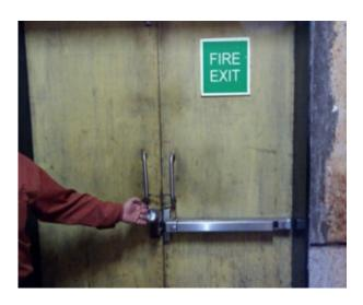
In a fire or other emergency, would you want to have to hunt for the key to the lock keeping you from using this fire exit'
