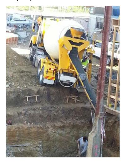
Various workplace, especially construction sites, feature trenches and excavations. Such digs pose several kinds of safety hazards, from cave-ins to hazardous atmospheres. This picture, which is from the Victorian WorkCover Authority (Australia), illustrates a few of those hazards.
