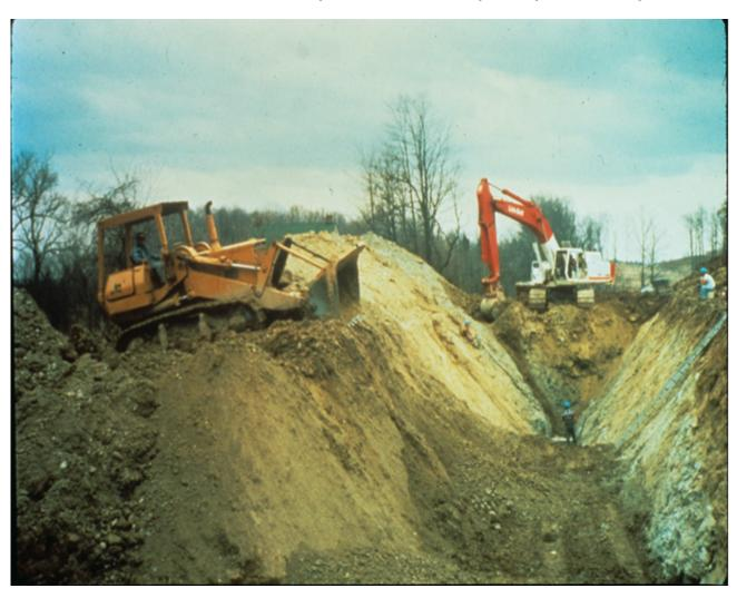
Trenches and excavations are very common in many workplaces, especially construction sites. They're also very hazardous. This picture from elcosh illustrates several of those hazards.
