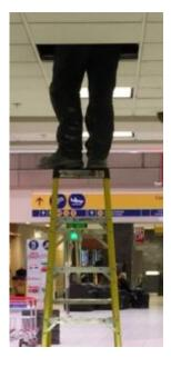
Is this worker properly'and safely'using a step ladder' What's he doing wrong'
