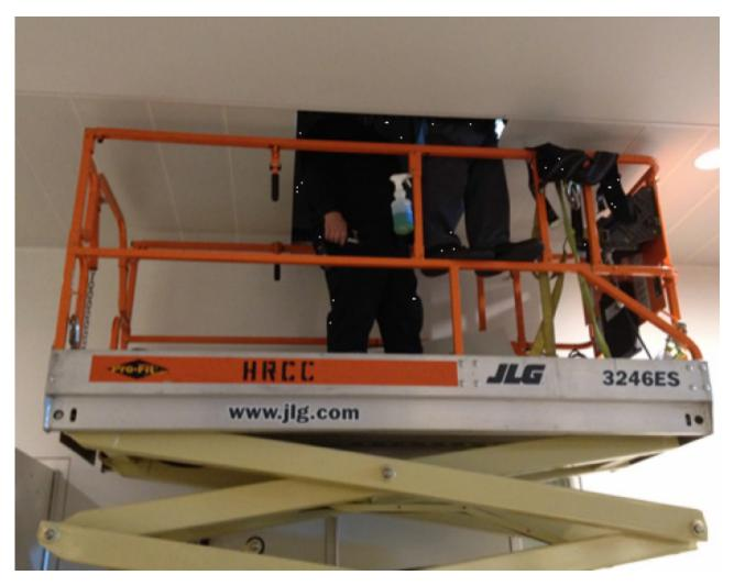
Improper use of scissor lifts can endanger workers. For example, in this picture from the Naval Safety Center, the worker shouldn't be standing on the side rail of the lift. These rails aren't intended to act as ladders. In addition, although there appears to be fall protection equipment on the scissor lift,
