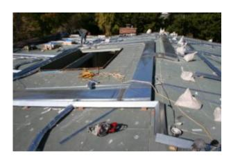
A crew for a roofing company removed heating, ventilation and air conditioning cones and other roofing material from the roof of an industrial establishment. The next morning, a worker fell through an opening in the roof and 28 feet to the concrete floor below, sustaining serious injuries. The company had failed to ensure that the worker was adequately protected by a guardrail system. It pleaded guilty and was fined \$57,500 [Paiva Roofing Ltd., Federal Govt. News Release, March 1, 2017].
