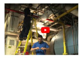
This WorkSafeBC video shows important safety procedures for ladder use in manufacturing, including setting up a stepladder, using one safely, and moving and positioning a ladder.
