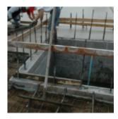
A worker was seriously injured when he fell through an opening in a floor and landed on a rebar dowel. His employer pleaded guilty to failing to ensure an opening at a worksite was securely covered and was fined \$10,500 [In 'N' Out Construction Inc., Govt. News Release, Feb. 9, 2016].
