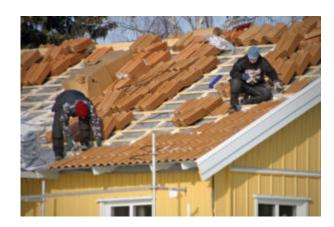
Seven workers were re-shingling the roof of a house without wearing any fall protection, even though they were working at a height of greater than three metres. In addition, there were no guard rails around the roof. Although no workers were injured, the roofing company was fined \$15,000 for failing to ensure that workers exposed to the hazard of a height greater than three metres were equipped with fall protection [Kelvin Chong Roofing Inc., Govt. News Release, Feb. 18, 2015].
