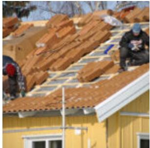
Seven workers were re-shingling the roof of a house without wearing any fall protection, even though they were working at a height of greater than three metres. In addition, there were no guard rails around the roof. Although no workers were injured, the roofing company was fined \$15,000 for failing to ensure that workers exposed to the hazard of a height greater than three metres were equipped with fall protection [Kelvin Chong Roofing Inc., Govt. News Release, Feb. 18, 2015].
