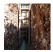
During an inspection of a worksite, an Occupational Health Officer saw workers working in a trench that wasn't properly shored and sloped. The employer pleaded guilty to failing to ensure that a worker present in a trench more than 1.2 metres deep was protected from cave-ins or sliding material and that all work at a place of employment was sufficiently and competently supervised. The court fined it \$9,800 [Empire Foundations Inc., Govt. News Release, May 30, 2014].
