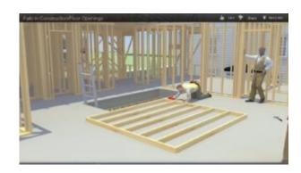
A worker was injured at the Carbon Capture Project at the Boundary Dam when he fell 15 feet through a hole in the floor of the worksite. His employer pleaded guilty to failing to ensure that any opening or hole in a floor, roof or other work surface into which a worker could step or fall was securely covered and/or protected. The court fined it \$10,000 [Sulzer Chemtech Canada Inc., Govt. News Release, July 10, 2014].
