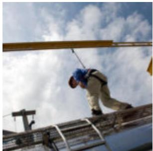
During the construction site of a long-term care facility, a steelworker fell approximately 15 feet from a steel joist, suffering head and wrist injuries. His employer was charged with two safety violations: failing to ensure that it provided and maintained a safe workplace and that a fall arrest system provided to a worker was adequately secured to an anchorage point or a lifeline [C. B. Metal Works Inc., Govt. News Release, Feb. 8, 2013].
