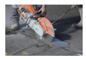
Two workers using gas-powered concrete saws to cut flooring in a retail space for the installation of plumbing systems were exposed to elevated levels of carbon monoxide and had to be taken to the hospital. The employer was convicted of 2 OHS offences for failing to protect the workers from exposure and fined \$120,000 [9819746 Canada Inc. operating as RENOCON, August 18, 2021].
