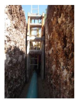
Two city workers were observed in a trench with straight cut sides and water seepage in the bottom. The walls of the excavation site didn't comply with OHS requirements. The city pleaded guilty to violating the OHS Act by failing to ensure that workers were protected from cave-ins or sliding materials in a trench and that all work was sufficiently and competently supervised. The court fined it \$6,180 [City of Meadow Lake, Govt. News Release, Aug. 7, 2012].
