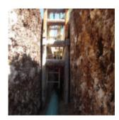
Two city workers were observed in a trench with straight cut sides and water seepage in the bottom. The walls of the excavation site didn't comply with OHS requirements. The city pleaded guilty to violating the OHS Act by failing to ensure that workers were protected from cave-ins or sliding materials in a trench and that all work was sufficiently and competently supervised. The court fined it \$6,180 [City of Meadow Lake, Govt. News Release, Aug. 7, 2012].
