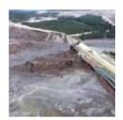
The Mount Polley Mine, operated by Imperial Metals, is an open-pit copper and gold mine near Likely, BC. It has a 4 km wide tailings pond built with an earthen dam that contains water and sand contaminated by various hazardous substances, including arsenic, lead and mercury.
