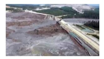
The Mount Polley Mine, operated by Imperial Metals, is an open-pit copper and gold mine near Likely, BC. It has a 4 km wide tailings pond built with an earthen dam that contains water and sand contaminated by various hazardous substances, including arsenic, lead and mercury.
