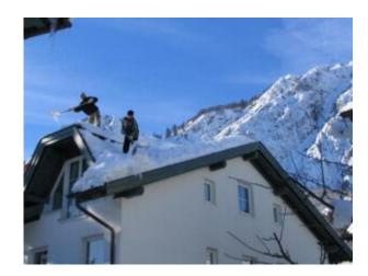
During the winter, snow and ice can build up on the roofs of your facilities. Their weight can damage the roof's structure and supports, and even lead to collapses.
